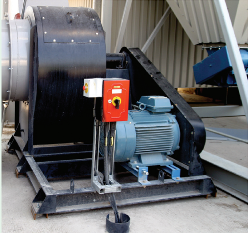
Halifax Beaufort 45kW exhaust fan.
