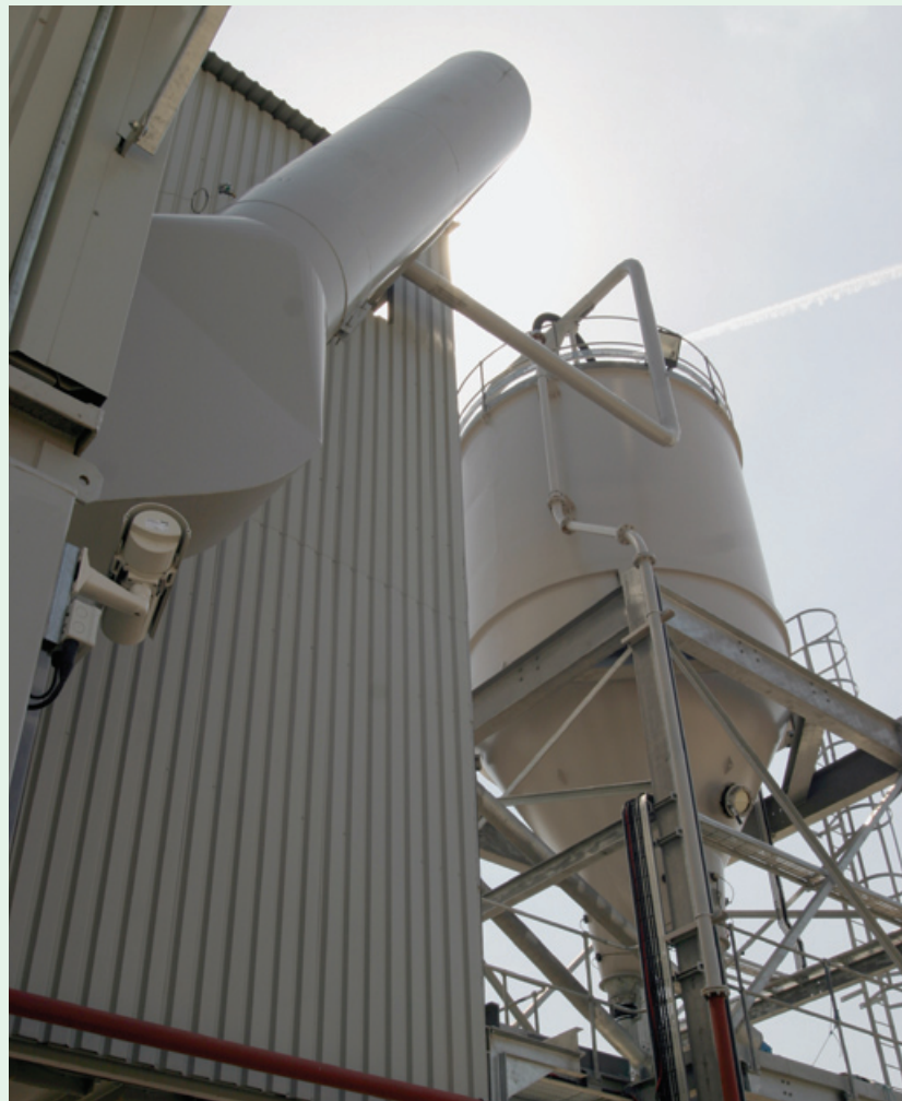
Mixlance Plant at Leeds delivers asphalt at 80 tons an hour
